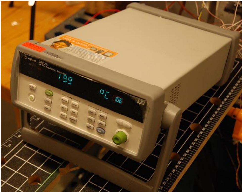
Fig. D.6. Agilent 34972A logging the voltage, current and inlet and outlet temperature, number 5 in figure D.1.
